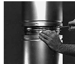
Step 3 Mate flanges of two pipes. Position Inner OVB over both flanges and tighten.
