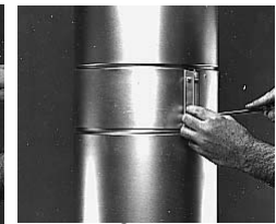
Step 4 Position Outer Channel Band around outer casing. Align with pipe grooves and tighten.
